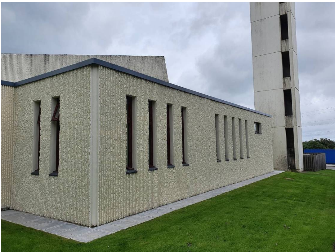
View of the right hand side of the extension
