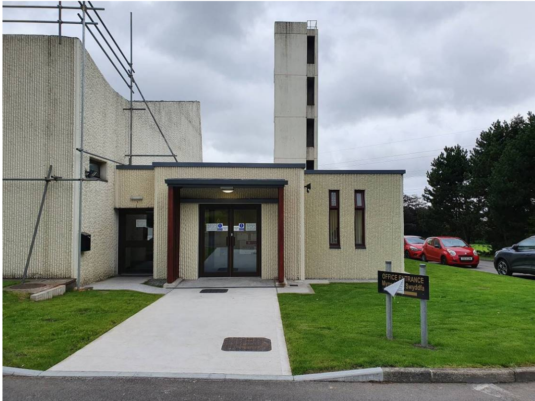
View of the front of the extension
